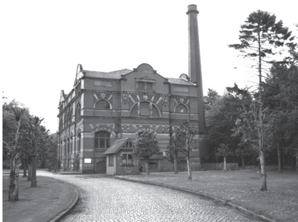
Boughton Pumping Station
